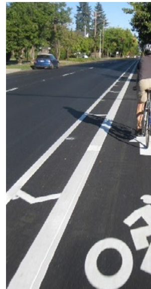
Buffered Bike Lanes. Photo courtesy of
